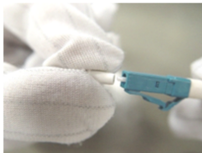
Figure 9-99 Installing a protective cap on a fiber
