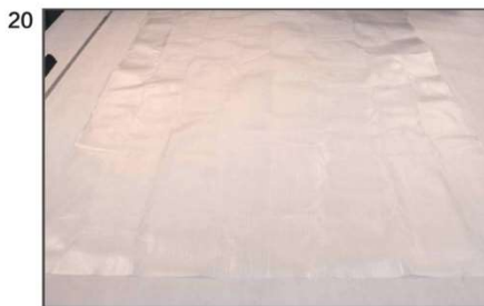
(20 Fabric install part: unfold the form on the ground,(flat ground))
